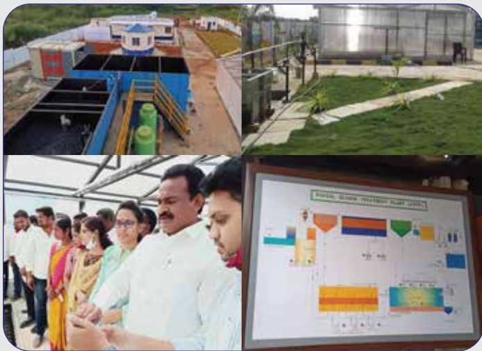
Facility was inaugurated by the Honourable MLA of Kamareddy, Sr. Gampa Govardhan garu on 18 th March, 2021.
